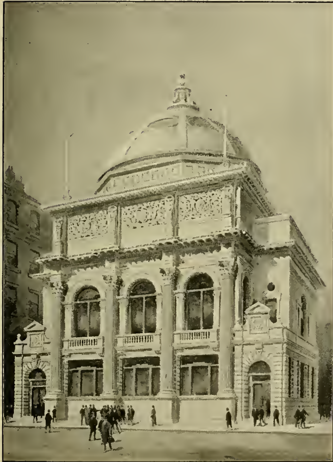
THE NEW YORK CLEARING HOUSE—Cedar Street, between Broadway and Nassan Street. R. W. GIBSON, Architect.
