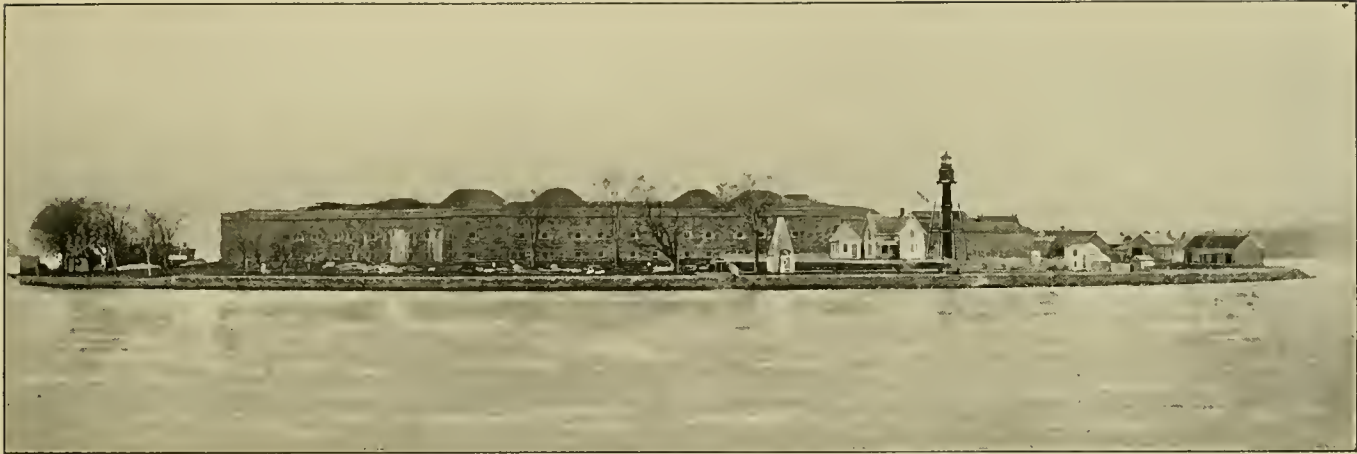
FORT SCHUYLER—Entrance to Long Island Sound.
