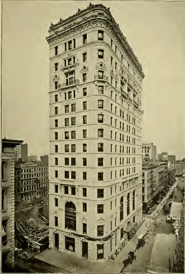
DUN BUILDING. Northeast Corner Broadway and Reade Street.
