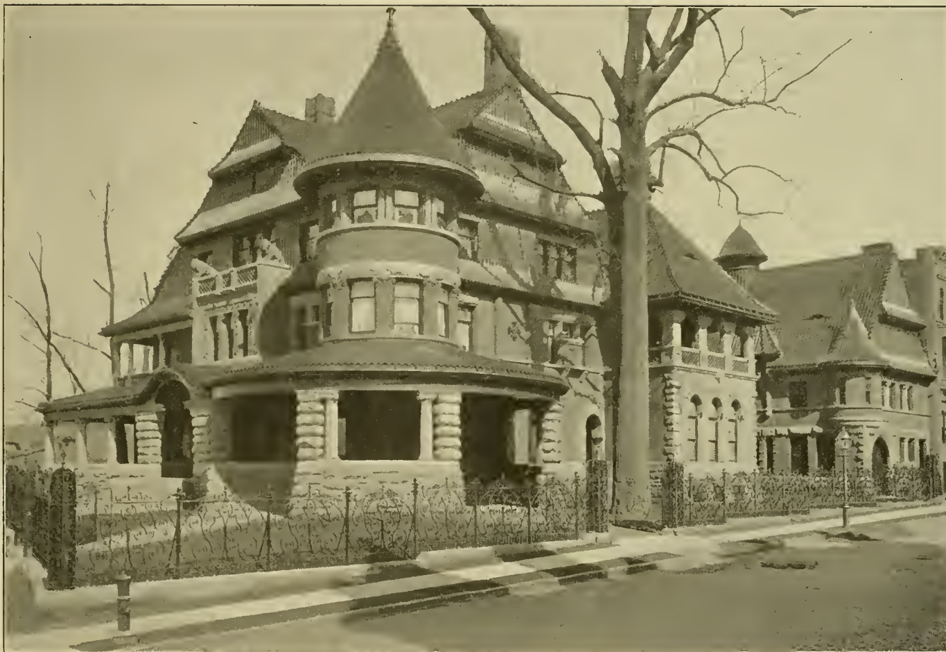
RESIDENCE OF JOHN H. MATTHEWS, ESQ.—Northwest Corner Riverside Drive and Ninetieth Street.
