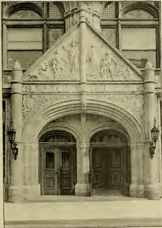
ENTRANCE, CHURCH MISSIONS HOUSE — Southeast Corner Fourth Avenue and Twenty-second Street. R. W. GIBSON, Architect.
